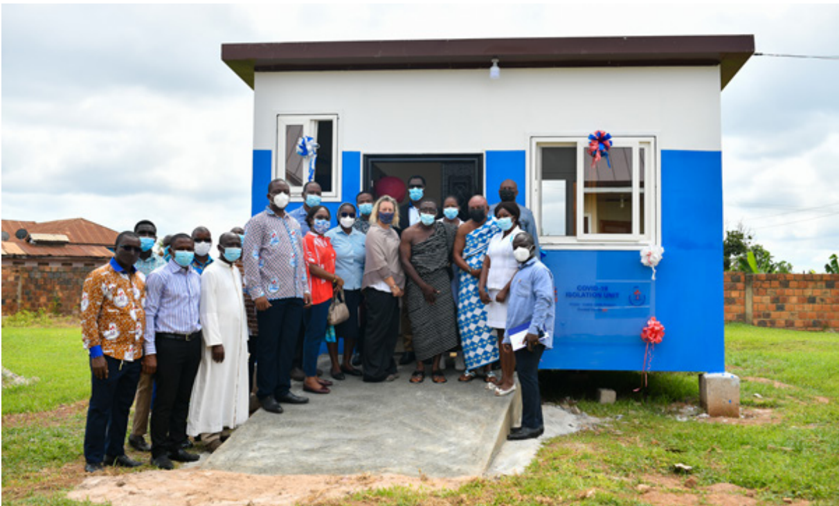
Figure 8: FIELD VISIT BY FCDO & CHAG HQ TEAM THE CRIB PROJECT SITES (ST ELIZABETH HOSPITAL ISOLATION UNIT AT HWIDIEM)
